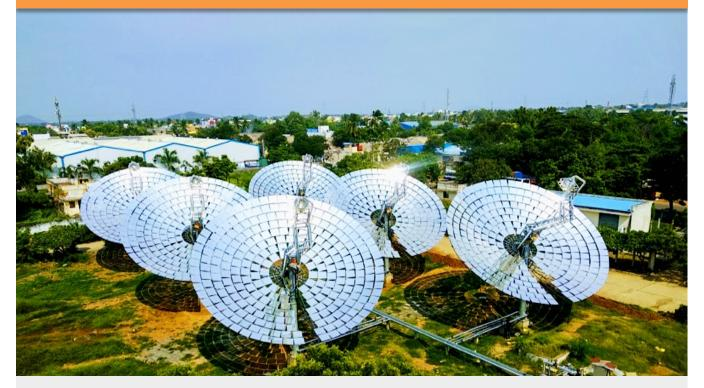
MWS SOLAR FIELD is a field of concentrating collectors designed to generate heat of a specific temperature and quantity for industrial process. Our technology-agnostic process allows us to deliver most optimal solution for customer based on variety of factors such as process, site specifics, radiation conditions etc. in form of various working fluids and upto 500°C
